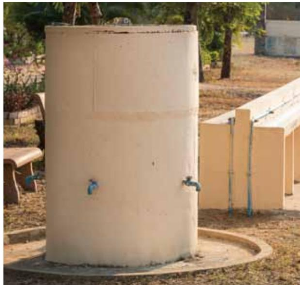
The tank in the photo on the right, made from stacked culverts, are able to accumulate enough water to ensure a year-round supply. This stood out in Cambodia for being the most impressive facility. It has to be stressed though that this facility was only made possible by the significant financial contribution of an individual donor.
