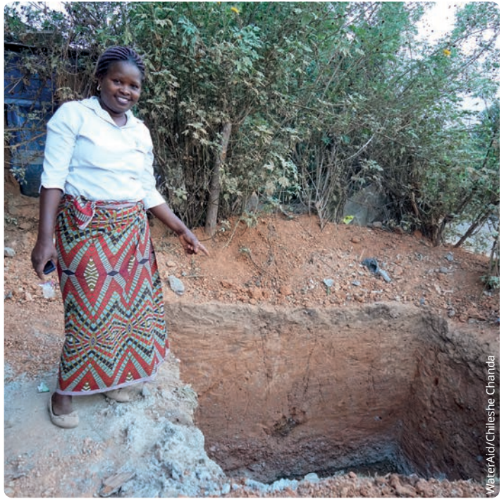
▲ Margaret, a resident of Kandeke Community, Ndola City, Zambia, shows the soak-pit for on-site sanitation at her house.
