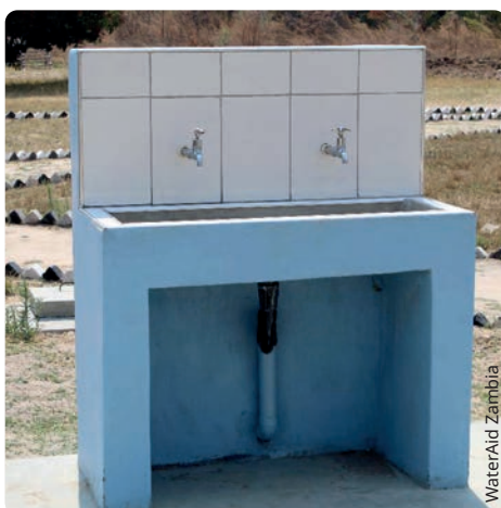
▲ HWF constructed in HCF in Zambia.
