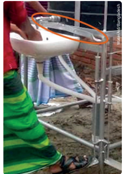
▲ A pedal working in a downward direction, but the lift cock is receiving an upward push through the lever action.
